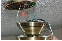
Insert two screws into the mounting plate, then lift the fan body onto the screws and secure it to the plate. Add a third screw if included by the manufacturer, and then slide the upper canopy in place.
