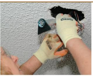
Install the hanger. After removing the old box, install the new. In this case, we used a fan-rated hanger bar and outlet box. The hanger bar is inserted first, squared up to the joists, and centered in the hole. The bar then is twisted clockwise, which pushes the barbed ends into the joists.
