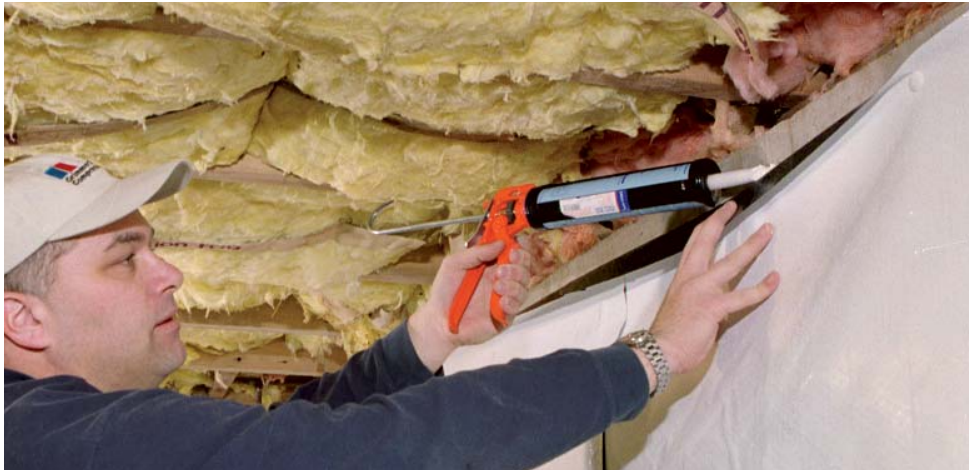
Seal the liner to the foundation with polyurethane caulk.
