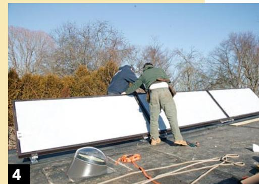
Solar hot-water systems involve a fair amount of labor-intensive planning and plumbing, but a typical collector installation is fairly straightforward. On this membrane-covered shed roof, **1** the first step was to erect the aluminum frames
