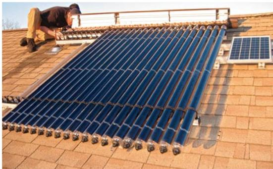
In these active systems, a pump circulates glycol in a closed loop. After running through high-efficiency evacuated-tube collectors (or flat-plate collectors), the hot glycol returns to the storage tank, where a heat exchanger warms potable hot water. Essentially freezeproof, these glycol-charged systems are able to perform in any season. Energyworks LLC in Portland, Maine, put the price of an installed system adequate for a local family of four at about \$10,000.
