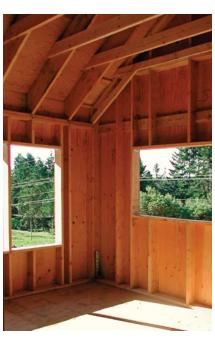
**Look!** No headers. Traditional framing (left) uses a lot of unnecessary wood. Optimum-value engineering (OVE; right) relies on careful structural analysis so that studs and headers are used only where they're needed. That means less wood, more insulation, and reduced thermal bridging.
