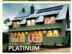
SIZE: 3200 SQ. FT. · Cost: \$230 per sq. ft. · Completed: 2006 · Bedrooms: 4, plus office · Bathrooms: 2½ · Location: Freeport, Maine · Architect: Richard Renner · Builder: Wright-Ryan Construction · Insulation: Walls, R-21 dense-pack cellulose; ceiling, R-49 loose-fill cellulose · Heating system: Radiant floor and woodstove · Cooling system: None · Windows: Thermotech triple-glazed; U-factor 0.15 · Green splurge: 2kw PV and solar hot water (\$30,000)
