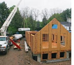
A crane provides muscle. Most of the time, walls can be tilted up by hand. However, for staging and stacking panels, tilting up large gable-end walls, and placing roof panels, a crane or a large forklift is a must.
