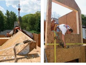
**Panels are moved into place with lifting plates and straps.** Steel lifting plates are screwed to the skin of wall and roof panels. Nylon webbing attaches to the pin on each plate. A crane or forklift grabs the webbing to move the panel where it needs to go. Manually operated ratchet straps have literally tons of pulling strength. Straps are essential for finessing large panels into difficult spots and for holding them in place while fastened.
