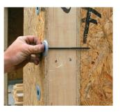
Electrocoated SIP screws with broad tin washers fasten the corner joints where dimensional lumber is installed. Midwall joints use splines that are slipped into channels routed in the foam. Splines are secured with 6d ring-shank nails; then expanding foam is inserted into the center channel to seal the joint.
