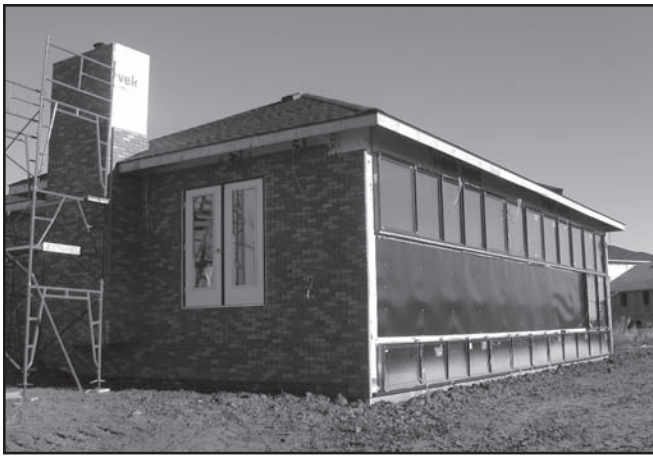
Figure 2. Most of the Factor 9 House windows face south. The two horizontal bands of south windows—one for the upper floor, and one for the lower floor—are separated by a band of vertical solar thermal collectors. This photo was taken after two of the home's 12 solar collectors had been installed. The height of the floor framing is indicated by the location of the door sill on the west side of the house.
