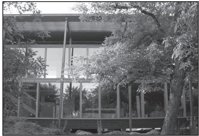
Figure 3. The designers of the S-House in Böheimkirchen, Austria, have described it as a Factor 10 house. Most of the building's glazing faces south.
