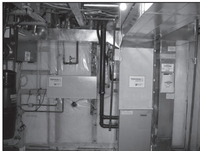
Figure 9. The RadiantLink box plenum is installed on top of a hot-air furnace. A separate wall-mounted box (the “control panel”) contains a circulator and an expansion tank.
