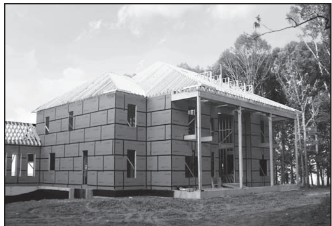
Figure 10. According to Huber Engineered Woods, a house sheathed with taped Zip System panels does not require housewrap or asphalt felt.
