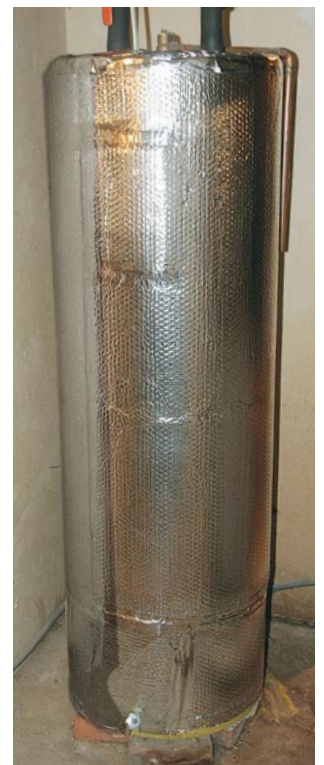
This insulation jacket from Energy Efficient Solutions ( www.energyefficientsolutions.com ) has an R-6 value and fits most tanks up to 80 gal.
