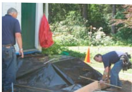
Contain paint chips at the edges. Turn the plastic edge up and support with lumber. Attach plastic to the house with furring strips, nails, and tape.
