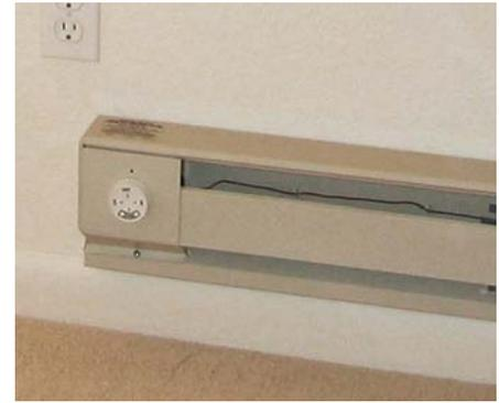
The heating element in an electric baseboard unit works just like the element in a toaster. Any electrician can install these units fairly quickly. The main drawback to this solution is that in most areas of the country, electric-resistance heat is expensive to operate. Still, electricity costs vary widely in the United States, from a low of about 6¢ per kwh to as much as 20¢ per kwh. The lower your electricity cost, the more attractive electric-resistance heating becomes.
