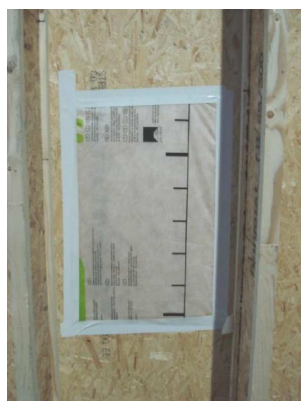
Figure 1: Ballooning of airtight foil on OSB surface during de-pressurization test
