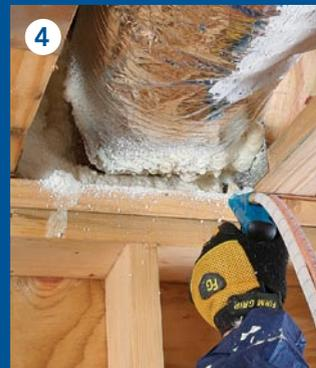
Foam expands to fill all gaps, holes, and joints susceptible to wood movement.
