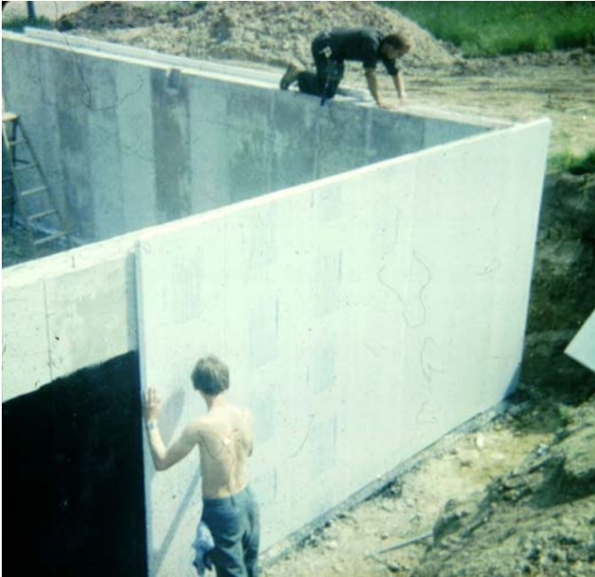
Photograph 1: Exterior Basement Insulation
