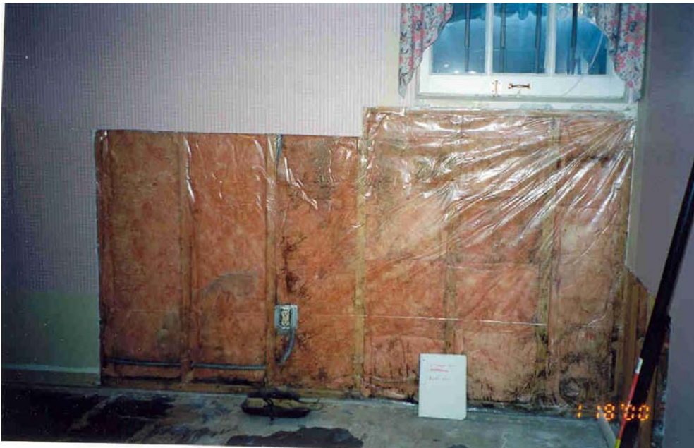
Photograph 2: Interior Frame Wall With Plastic Vapor Barrier
