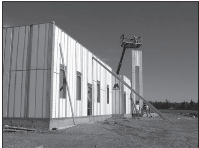
Figure 7. Nascor wall panels have embedded wood I-studs with OSB webs.
