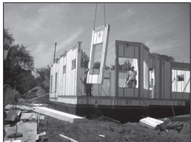
Figure 5. Most Energy Wise wall panels are four feet wide.
