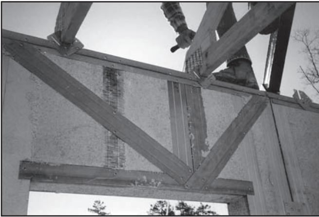
Figure 8. The ThermaSteel wall panels at this house are joined by a steel top plate.
